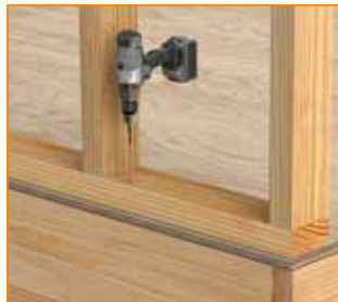
BOTTOM PLATE TO RIM BOARD
