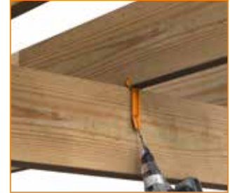
BEAM TO JOIST
