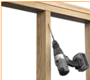
STUD TO DOUBLE TOP PLATE
