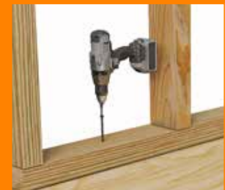
BOTTOM PLATE TO FLOOR JOIST
