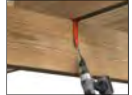
DECK JOIST TO BEAM
