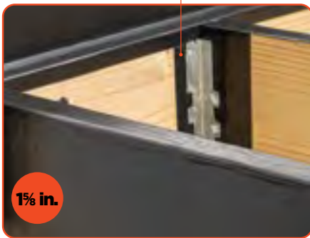
A BETWEEN JOIST HANGERS AND LEDGER BOARD
