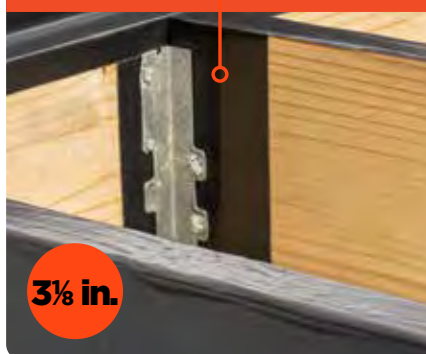
BETWEEN FRAMING AND JOIST HANGERS
