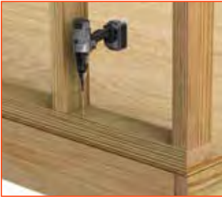
BOTTOM PLATE TO RIM BOARD
