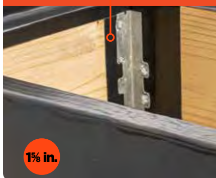
BETWEEN JOIST HANGERS AND LEDGER BOARD
