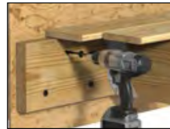
LEDGER BOARD CONNECTIONS
