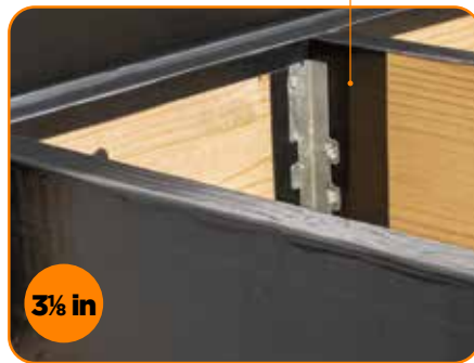
B BETWEEN FRAMING AND JOIST HANGERS
