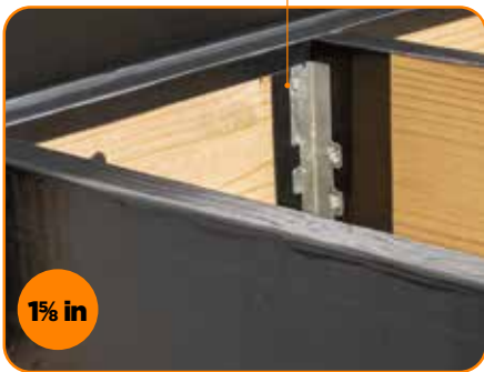
A BETWEEN JOIST HANGERS AND LEDGER BOARD
