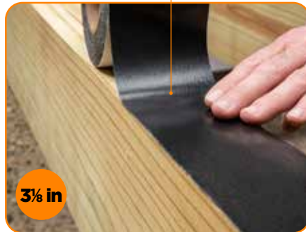
E TOP OF DOUBLE JOISTS
