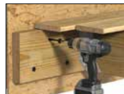
LEDGER BOARD CONNECTIONS
