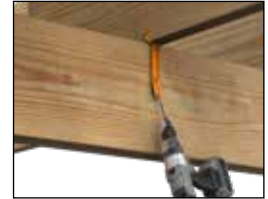
DECK JOIST TO BEAM
