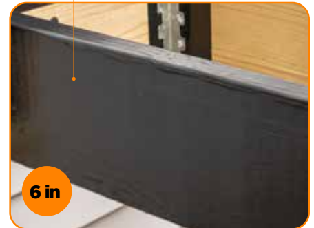
F BETWEEN RIM JOISTS AND FASCIA
