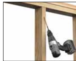
STUD TO DOUBLE TOP PLATE
