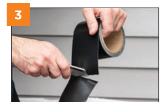
3 CUT TAPE TO THE DESIRED LENGTH
