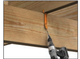
DECK JOIST TO BEAM
