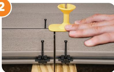
Place the next board up against the clips then fasten the screws.
