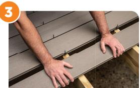
Slide the next board up against the clips, and repeat until you have multiple rows of boards and clips.
