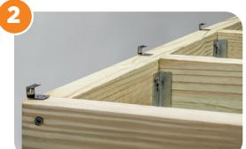
Repeat to install a clip at every joist. Do not skip any joists.
