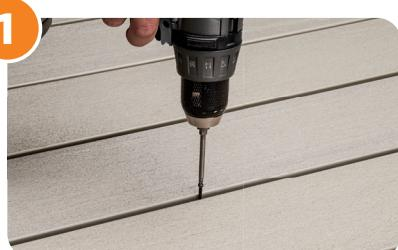
Back out all of the screws from the joist on both sides of the board.
