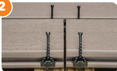
With boards positioned correctly, place the clips in the groove, centered on joists on both sides of the boards. Partially fasten the screws to hold them in place until next board is set, then fully fasten the screws.
