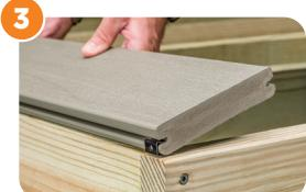
Tilt the deck board up slightly to set it in the clips.
