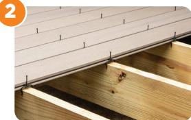
Place a clip at every joist along the length of the board.
