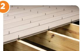
Install a clip at every joist along the length of the board.
