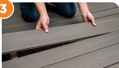
Clean away any clips remaining on the joists and lay the new deck board in position without any clips in place.
