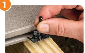
Tilt the WEDGE Clip so the lower prongs enter the groove first. Tilt the clip back up to wedge into the groove. Clips stay in place until you're ready to fasten.
